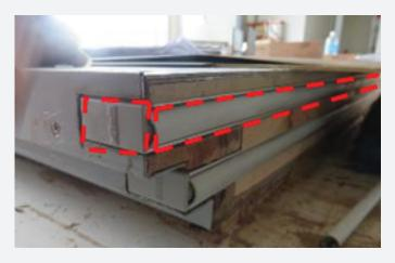
To cut the groove (highlighted in red) for installing bottom panel of timber door frames
